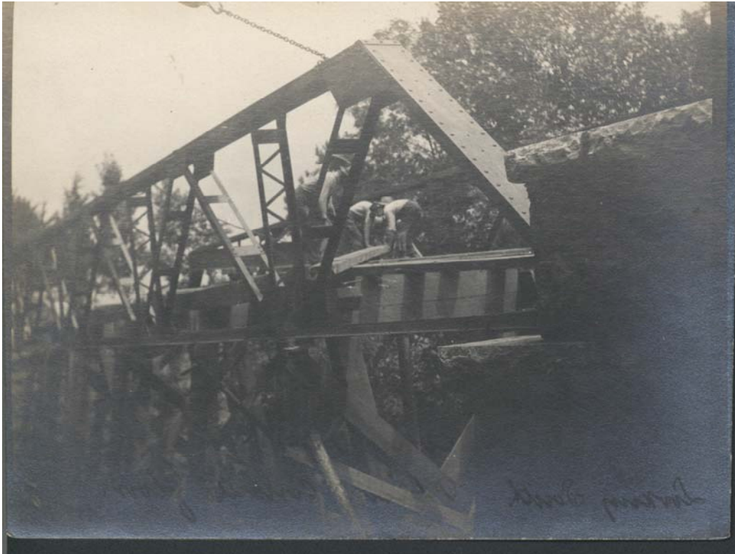
Figure 5. Alexander's Bridge under construction, August 1907.
