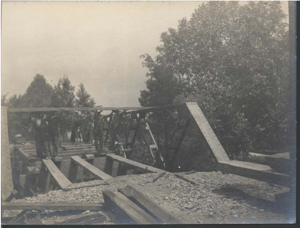
Figure 6. Alexander's Bridge trusses in position preparatory to riveting together, August 1907.
