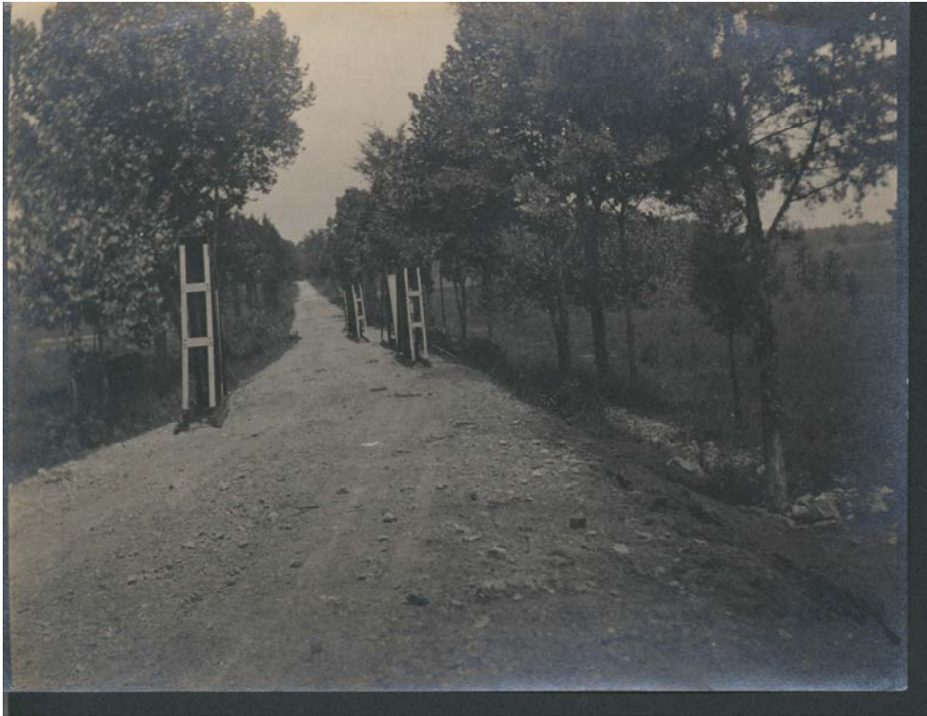
Figure 3. Partially assembled truss members delivered to site of Alexander's Bridge, August 1907.
